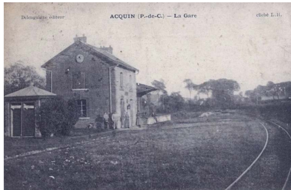
Acquin station around 1910: to the left we can see the toilets and lamp house (postcard, coll. CCHP).
