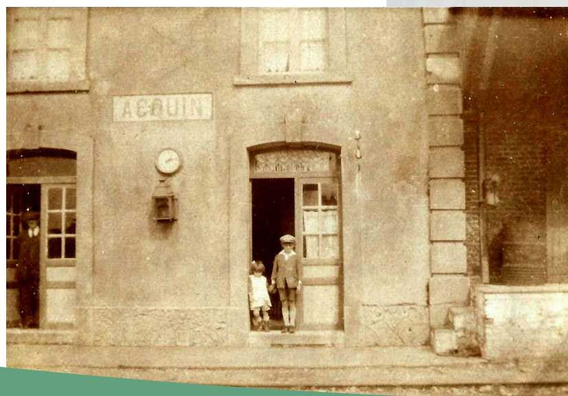
Odette and Roger Météyer in front of Acquin station, around 1935. The warehouse can be seen to the right (coll. Arnauld Météyer).
